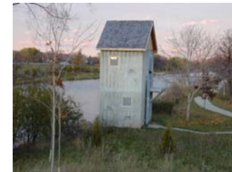
Continuous Dissolved Oxygen Monitoring Station
